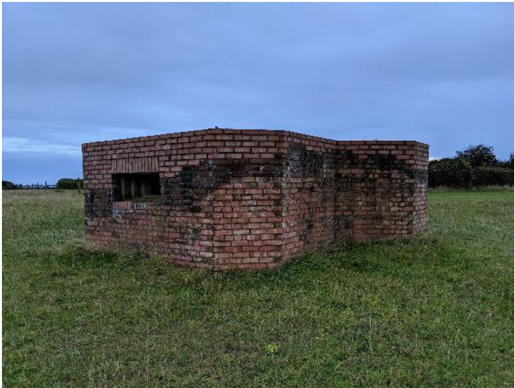
Plate 21.1.4-27 View of southern face of pillbox, looking north.
