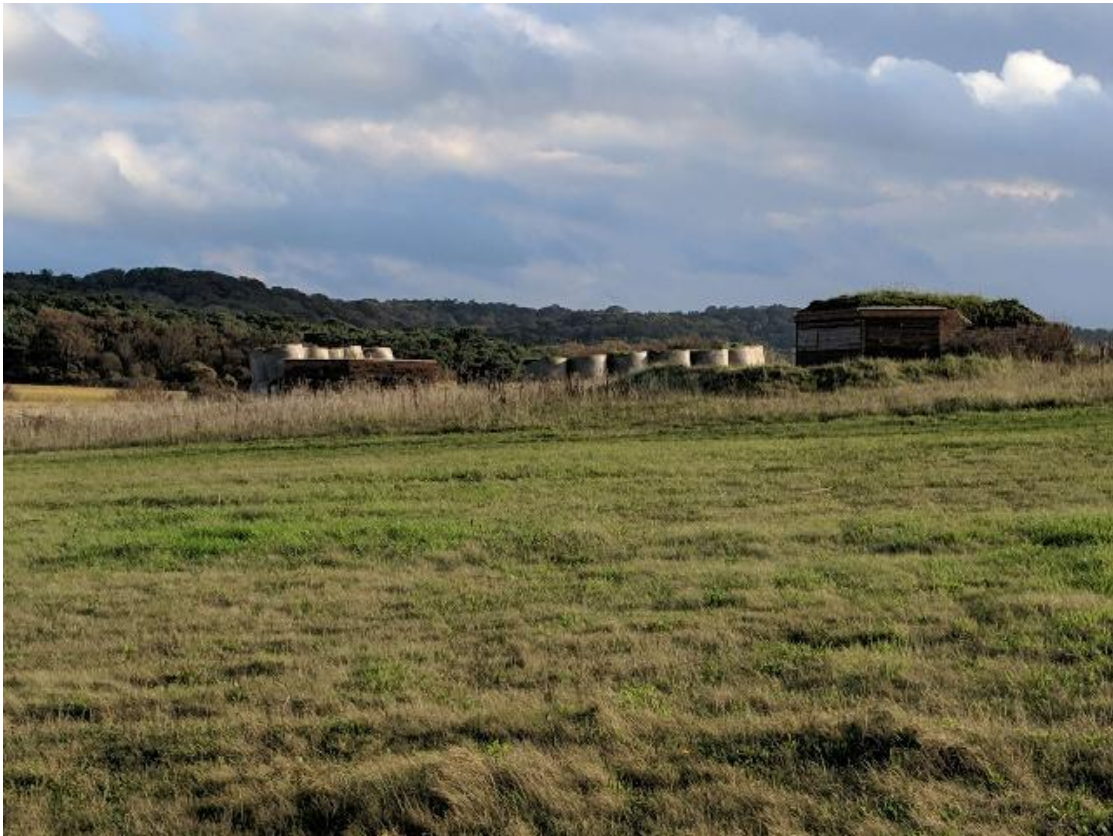
Plate 21.1.4-32 View from the north, along Norfolk coastal walk, looking south towards the pillboxes.
